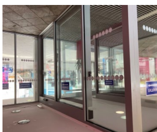
New Front Entrance
